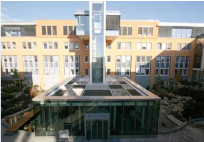
Company headquarters in Wiesbaden
