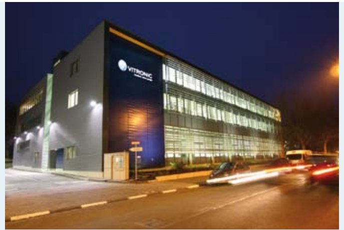
Production building in Wiesbaden
